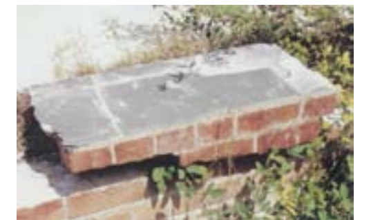
The image above shows a thin layer of slate used as a damp-course to prevent the upward movement of moisture.
