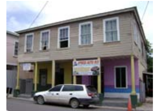
This commercial building on Market Street possesses a masonry ground floor and timber frame second story.
