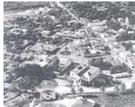
Aerial view of Market Street and Water Square.
