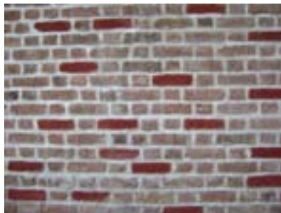
A brick building recently repointed with an historically appropriate lime mortar.
