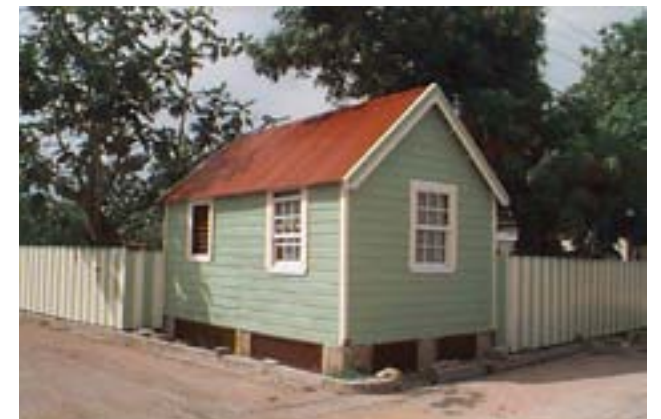
Above: A shingle roof was used in the rehabilitation of 31 Duke Street, which would have matched the original. A decorative cap-n-comb was also added to accentuate the style and character of the house. Below: A new corrugated metal roof was used in the rehabilitation of 7 Queen Street, which is consistent with the guidelines.
