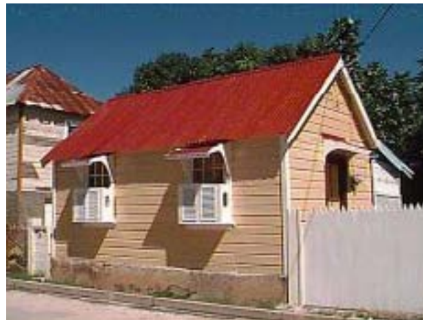
The restored coolers at 36 Cornwall Street are in keeping with the guidelines addressing windows restoration for historic structures in Falmouth.
