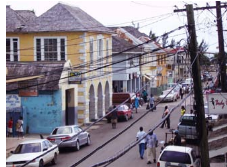
The overhead utilities along Market Street detract from the overall appearance of the street and its historic integrity.
